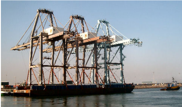
Figure 6: Barge Western Carrier departing Long Beach with 3 old cranes transversely stowed on deck
