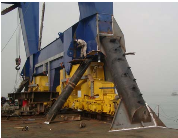
Figure 8: Pipe bracings fix crane corners to the deck
